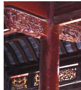
Fig.265. Detail of the queti design in the interior of the reception hall, Jingjue Mosque, Nanjing.
