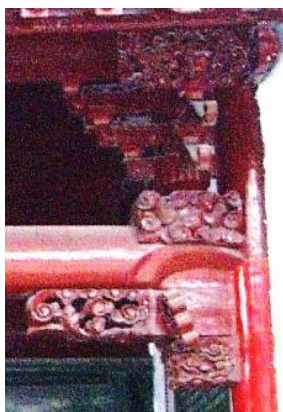
Fig.262. Detail of the wood carvings of the eastern entrance passage, Xianhe Mosque, Yangzhou.
