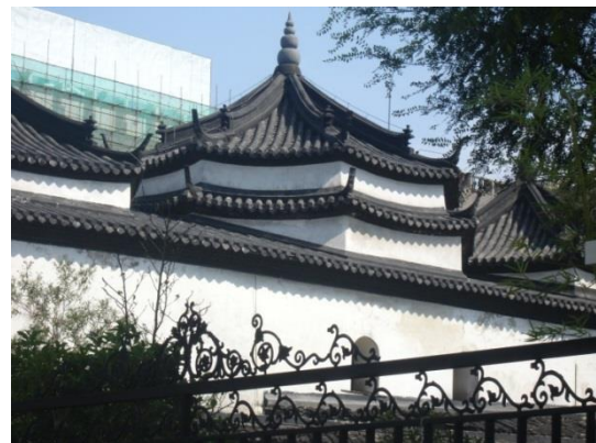
Fig.182. Elevated roof of the domed mihrab chamber of the Fenghuang Mosque, Hangzhou.
