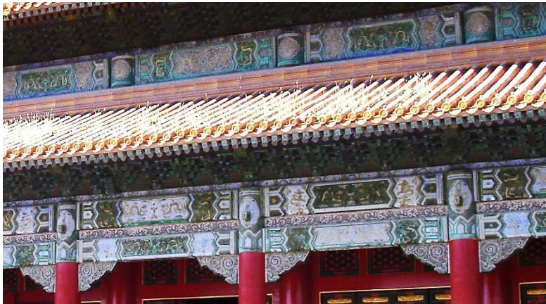
Fig.257. Detail of the decoration of the efang , dougong and queti of the Taihedian in the Forbidden City, Beijing.
