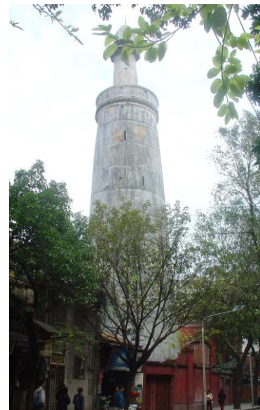
Fig.140. Guangta Minaret, Huaisheng Mosque, Guangzhou.
