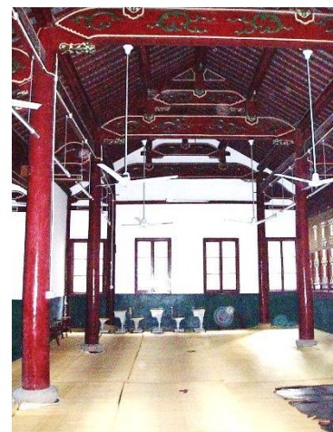
Fig.109. Interior of the prayer hall, Fuyoulu Mosque, Shanghai.
