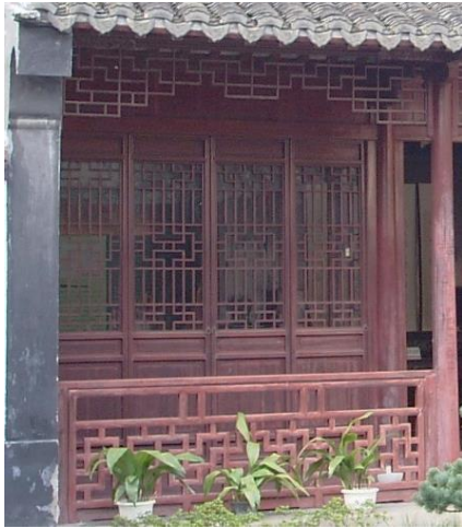
Fig.242. Balustrade at the balcony of the teaching hall, Songjiang Mosque, Songjiang.
