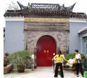
Fig.98. Front elevation of the south entrance, Luhe Changjianglu Mosque, Nanjing.
