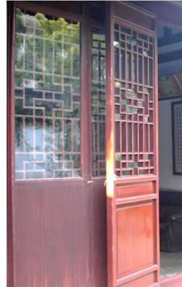
Fig.248. Screen doors of the reception hall, Songjiang Mosque, Songjiang.
