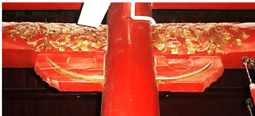
Fig.267. Detail of the painted beam and the queti in the prayer hall, Jiaxing Mosque, Jiaxing.
