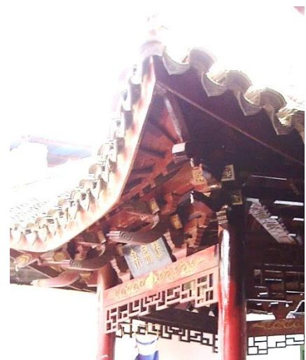
Fig.261. Detail of the dougong brackets of the pavilion, Jiaxing Mosque, Jiaying.
