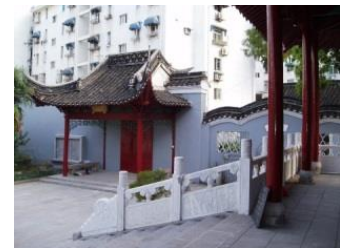
Fig.99. Back elevation of the south entrance, Luhe Changjianglu Mosque, Nanjing.
