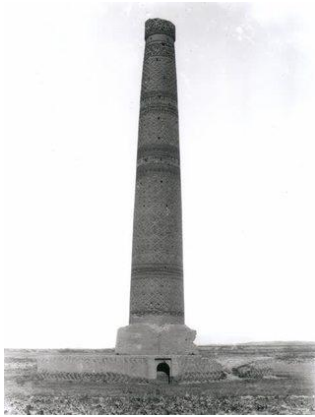
Fig.137. Minaret in Khosrawgird, Sabzavar, Iran. (From http://archnet.org/sites/5491 )
