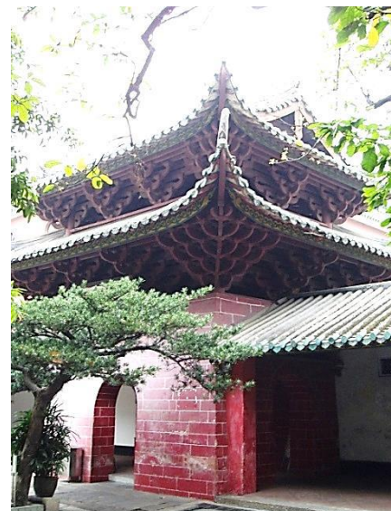
Fig.71. Entrance gateway as the wanyue lou , Huaisheng Mosque, Guangzhou.
