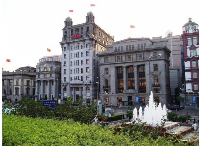
Fig.121. View of the colonial buildings in the former foreign concession, Shanghai.
