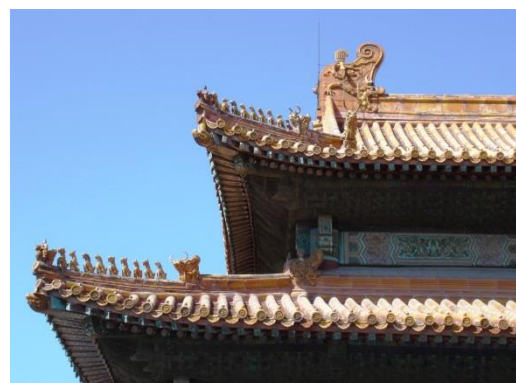
Fig.172. Roof-figures of the Baohedian in the Forbidden City, Beijing.
