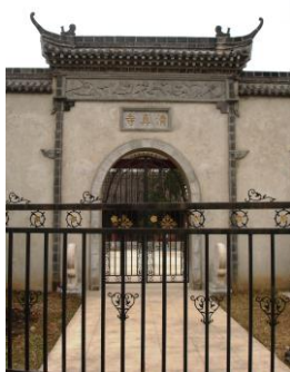
Fig.63. Front elevation of the east entrance gate, Luhe Nanmen Mosque, Nanjing.
