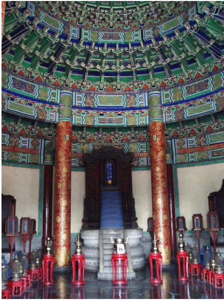
Fig.19. Zhaojing ceiling of the Qiniandian, Tianan, Beijing.
