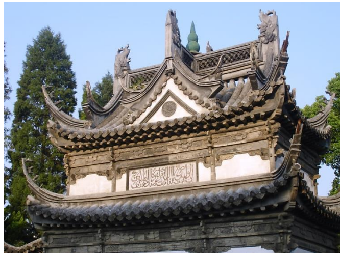
Fig.183. Roof of the minaret of the Songjiang Mosque, Songjiang.
