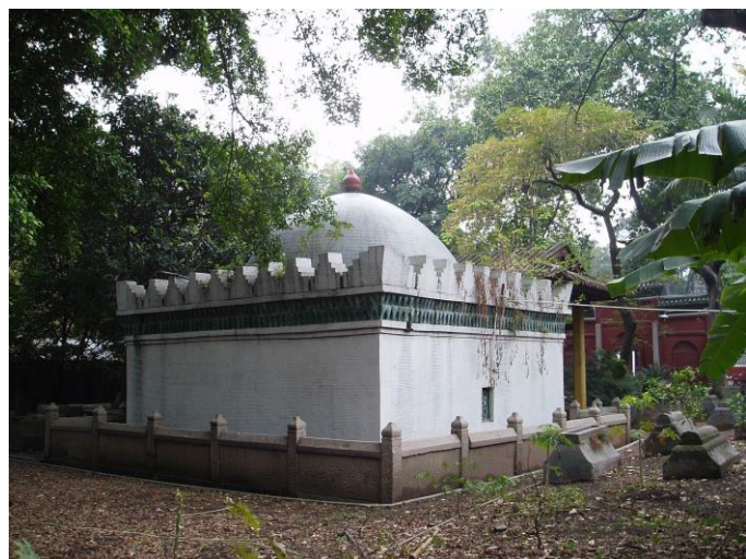
Fig.23. Elevation of the tomb of Sa'd Ibn Abi Waqqâs, looking southwest, Guangzhou.
