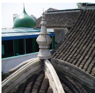
Fig.155. Detail of the pyramidal roof of the wangyue ting , Jiaxing Mosque, Jiaxing.
