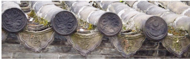
Fig.185. Detail of eaves-tiles, Baha al-Din tomb complex, Yangzhou.
