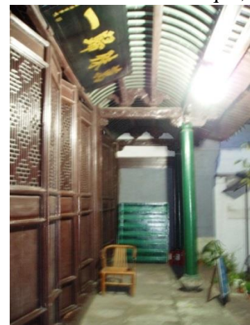
Fig.76. Balcony of the prayer hall, Ningbo Mosque, Ningbo.
