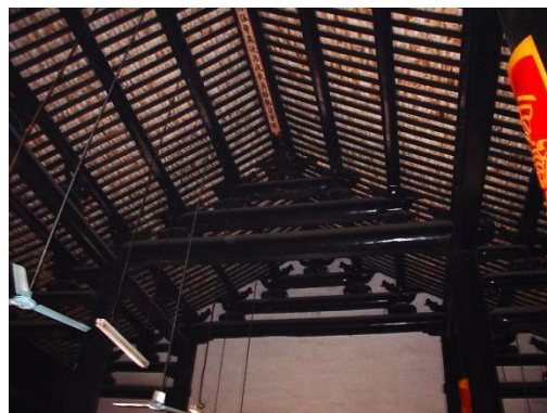
Fig.70. Interior of the prayer hall, Haopan Mosque, Guangzhou.
