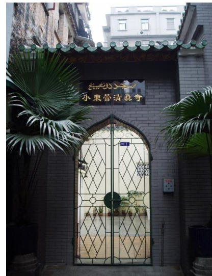
Fig.51. Entrance gate, Xiaodongying Mosque, Guangzhou.
