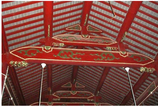
Fig.269. Painted beams in the prayer hall, Fuyoulu Mosque, Shanghai.
