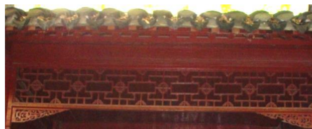
Fig.259. Detail of the decorative screen of the efang of the western entrance passage, Shanxiang Mosque, Zhenjiang.
