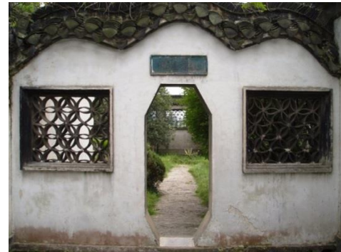
Fig.208. Garden enclosure, showing a dongmen and flanking louchuang , Baha al-Din tomb complex, Yangzhou.
