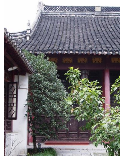
Fig.54. Xieshan roof of the prayer hall, Jingjue Mosque, Nanjing.
