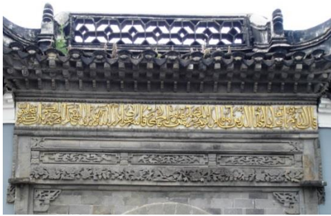
Fig.203. Decoration on the entrance gateway, Luhe Changjianglu Mosque, Nanjing.
