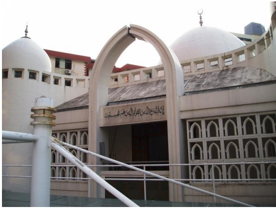
Fig.119. Elevation of the upper storey of the prayer hall, Huxi Mosque, Shanghai.
