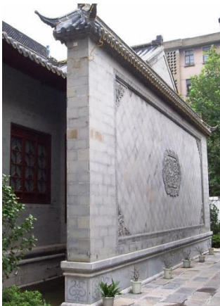
Fig.200. Screen wall, Caoqiao Mosque, Nanjing.
