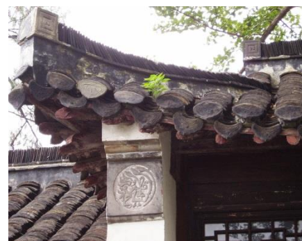
Fig.198. Inscription on an eaves wall, Baha al-Din tomb complex, Yangzhou.
