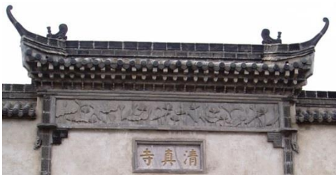
Fig.204. Decoration on the entrance gateway, Luhe Nanmen Mosque, Nanjing.
