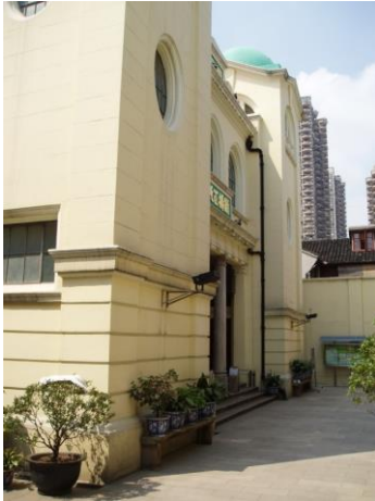
Fig.124. Front elevation of the prayer hall, Xiaotaoyuan Mosque, Shanghai.
