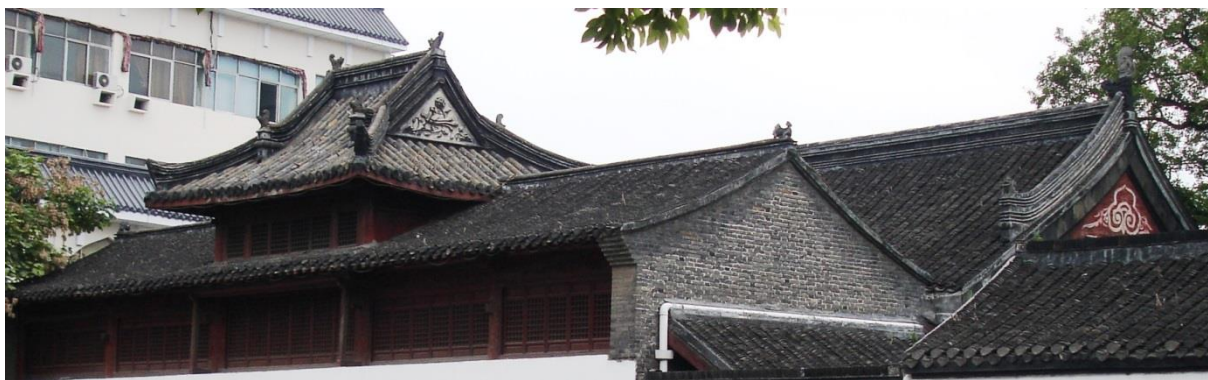
Fig.189. View of the roof of the prayer hall, Xianhe Mosque, Yangzhou.
