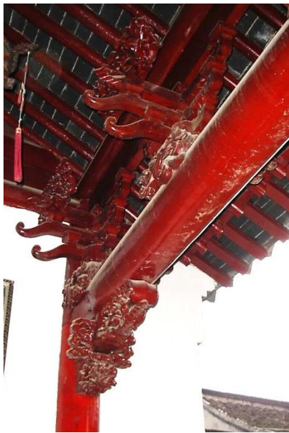
Fig.260. Detail of the decoration of the dougong and queti brackets of the Eastern entrance passage, Xianhe Mosque, Yangzhou.
