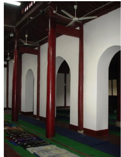
Fig.88. Interior of the prayer hall, showing the partition wall, Xianhe Mosque, Yangzhou.
