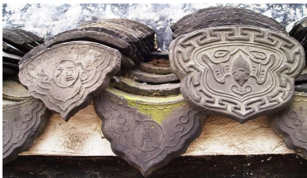
Fig.188. Detail of eaves-tiles, Baha al-Din tomb complex, Yangzhou.
