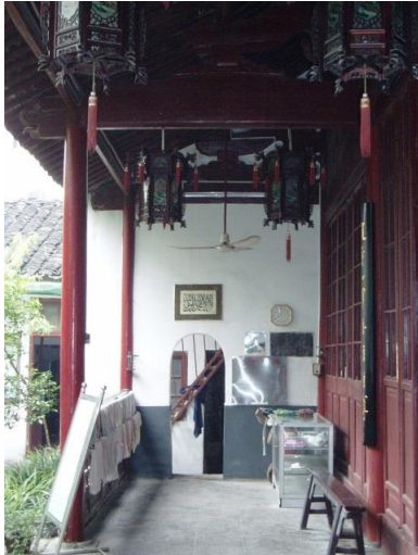
Fig.117. Balcony of the prayer hall, Jizhaoying Mosque, Nanjing.
