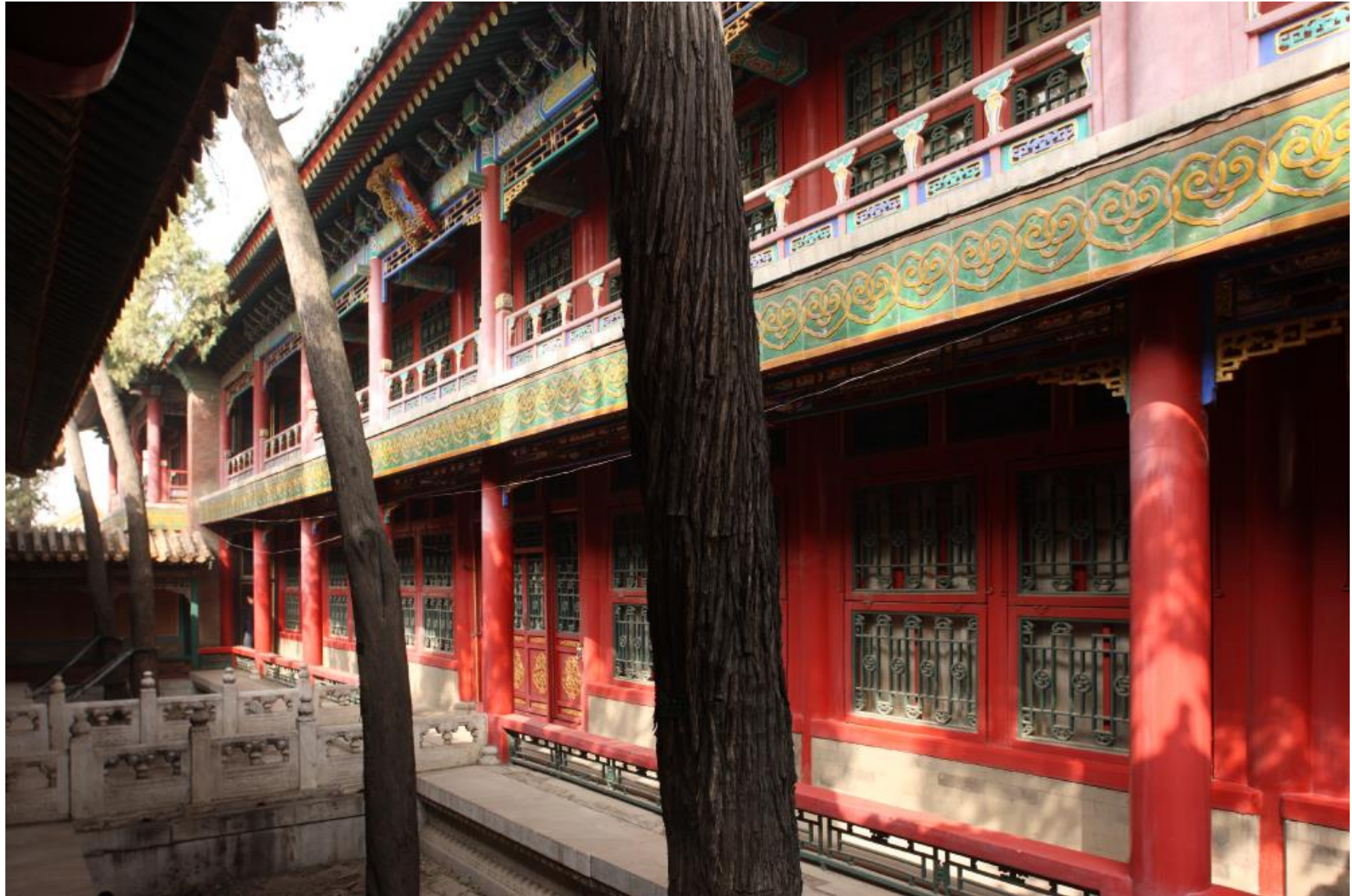
Fig.2.1 The exterior of Fanhualou. After "梵华楼 = Fanhualou.", dpm.org.cn , Accessed 1 September 2023, https://www.dpm.org.cn/explore/building/236572.html .
