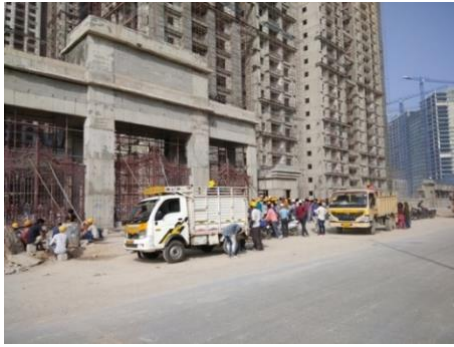
Figure 7.1: Labourers waiting to enter a construction site at 8.30 am
