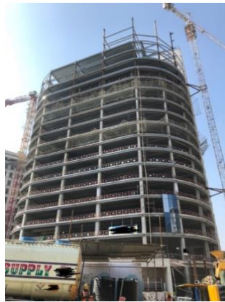
Figure 6.4: Construction Site B (BSS)
