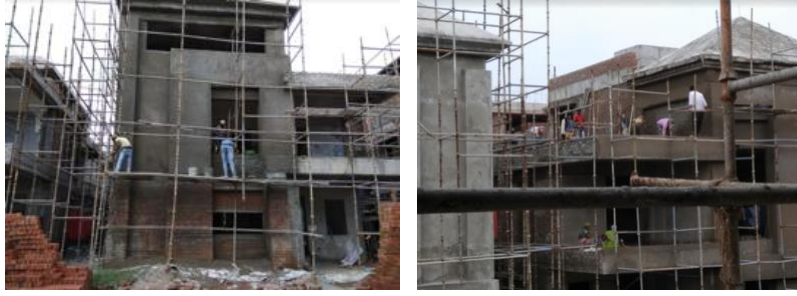
Figure 6.2: Masonry work at Rishabh's site (Source: Photographed by the author, 2019)
