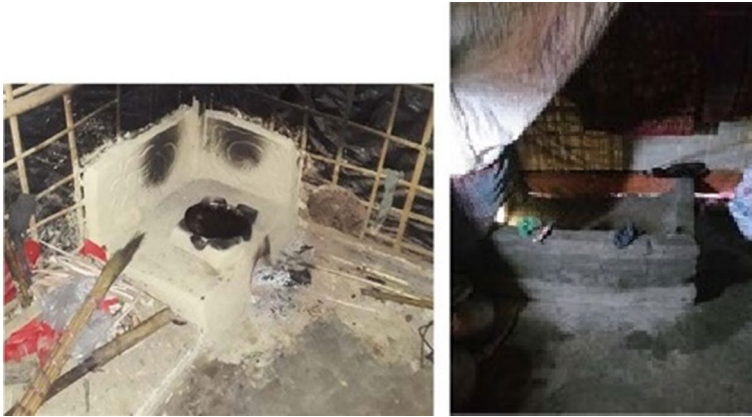
Fig. 12 left: Cooking area protected by small mud walls. The proximity of the flammable plastic tarpaulin and bamboo is evident. Right: Typical self-built in-shelter bathing area found
