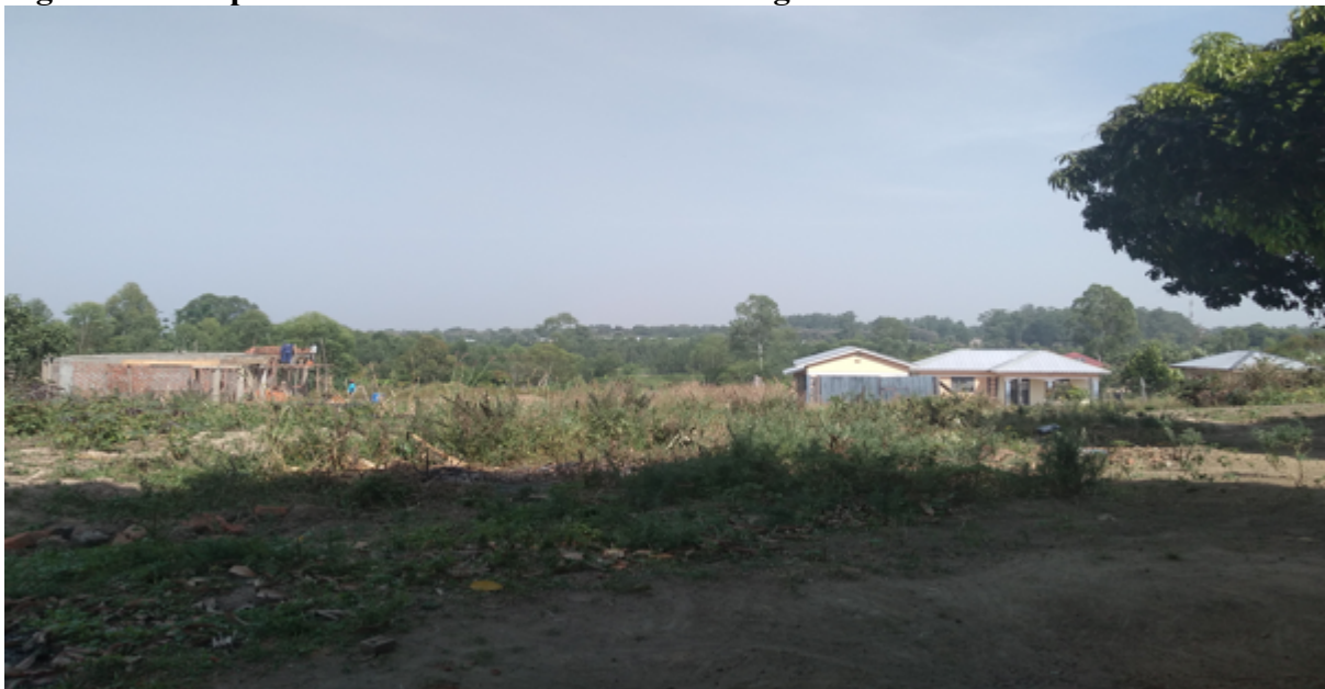
Figure 20. Joseph's home under construction among other South Sudanese homes
