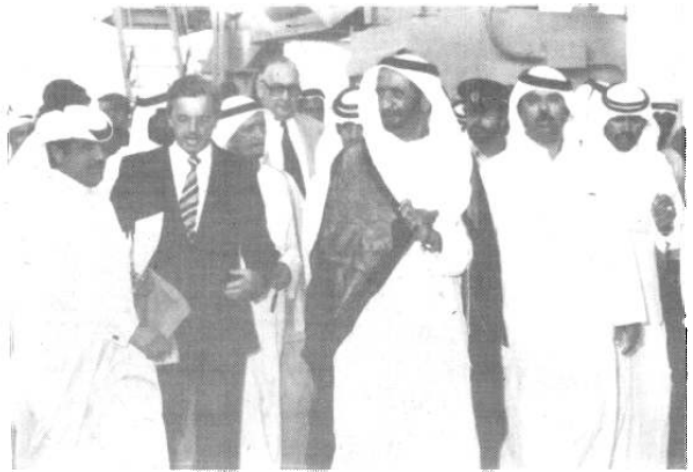
Sheikh Rashid, accompanied by Port Rashid's Captain Butcher (in dark suit) and other distinguished invitees tours the new container terminal yesterday.—Gulf News photograph.
