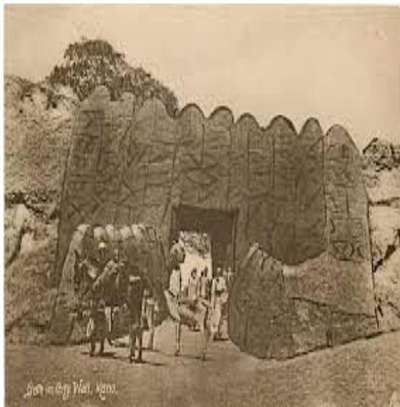
Fig.21: Kano City Wall (1922)
