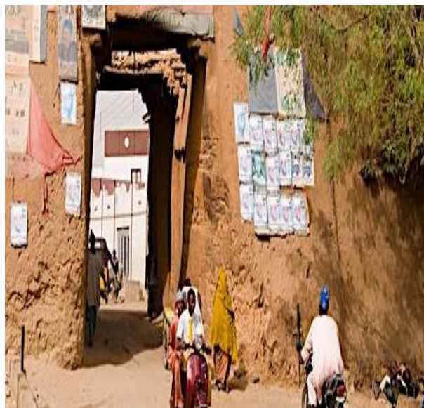
Fig.22: Kano City Wall – (2018)
