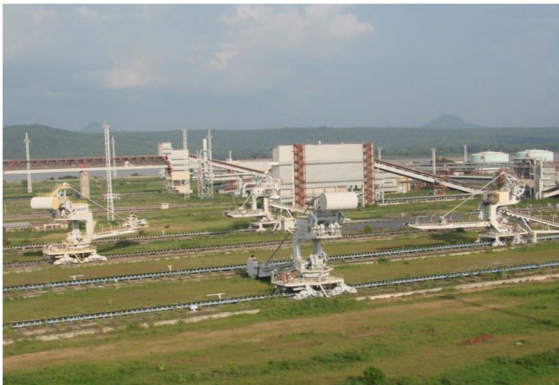
4: Ore and fluxes stockyard with stackers and reclaimers (100% completed)
