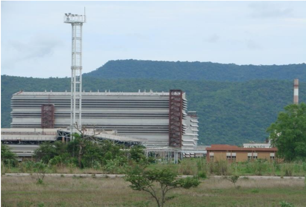
23: Alumino-Silicate refractory plant (to be used in industrial furnaces of still plant, oil refineries, cement factories etc; capacity, 43, 400 tons/year (Alumino-silicate refractory bricks))
