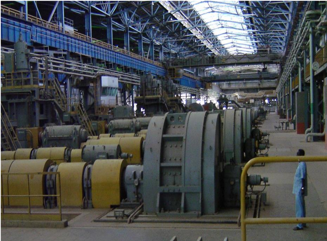
18: Medium section and structural mill (100% completed)
