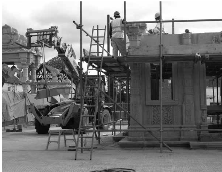
9 Construction of the Shiva shrine at the Sanatan Hindu Mandir, Wembley, London, 2011.
