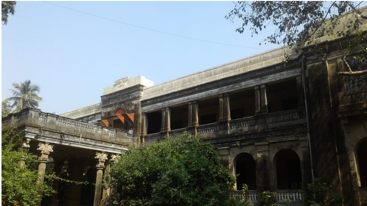
Figure 7: The M. F. Cama Athornan Institute building in Andheri, Mumbai
