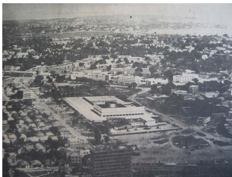
Fig. 1.25 The planned Mnazi Mmoja Parliament. In 1967 London architects Anthony R. Davies & Partners designed a new Parliament, planned for construction on Mnazi Mmoja. It had been anticipated that envisaged costs of £1,000,000 were to be met mostly from a British Government loan. However, the loan was frozen after Britain-Tanzania relations were suspended in 1965 and no alternative source of funds appears to have been identified as the Parliament was never built.
