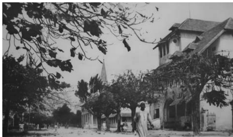
Fig. 1.14 Post Office, Main Avenue (1929)
