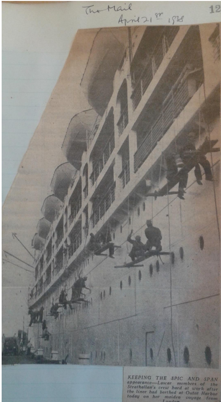
Lascars suspended from 'floating stages' painting the sides of the ship. (P&O/98/67, National Maritime Museum, Greenwich.)
