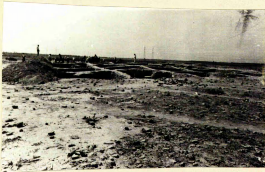
b. View showing general excavations in Area 'B' .
