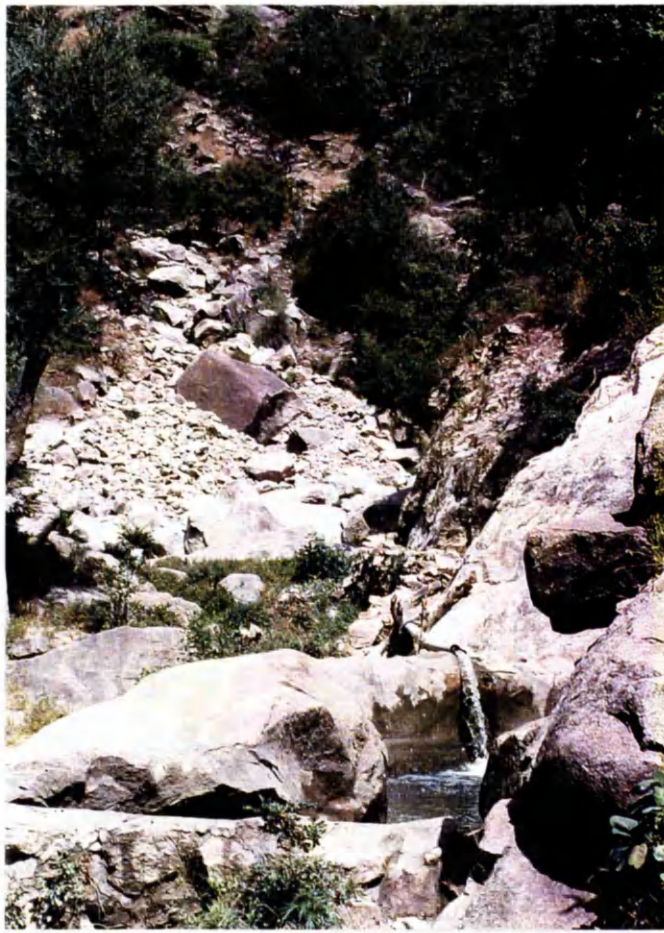
Photo 3: Water Diversion Structure Tapping Sub-Surface Wadi Flow. Wadi Nibaq irrigation source.
