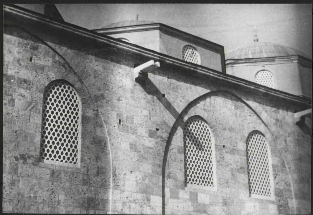
FIG. 37 THE FACADE OF THE BURSA ULU CAMI
