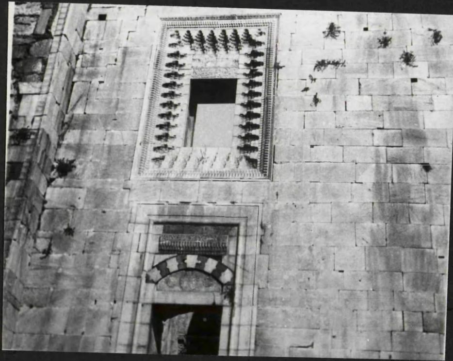
FIG. 20 THE FACADE OF İSA BEY
