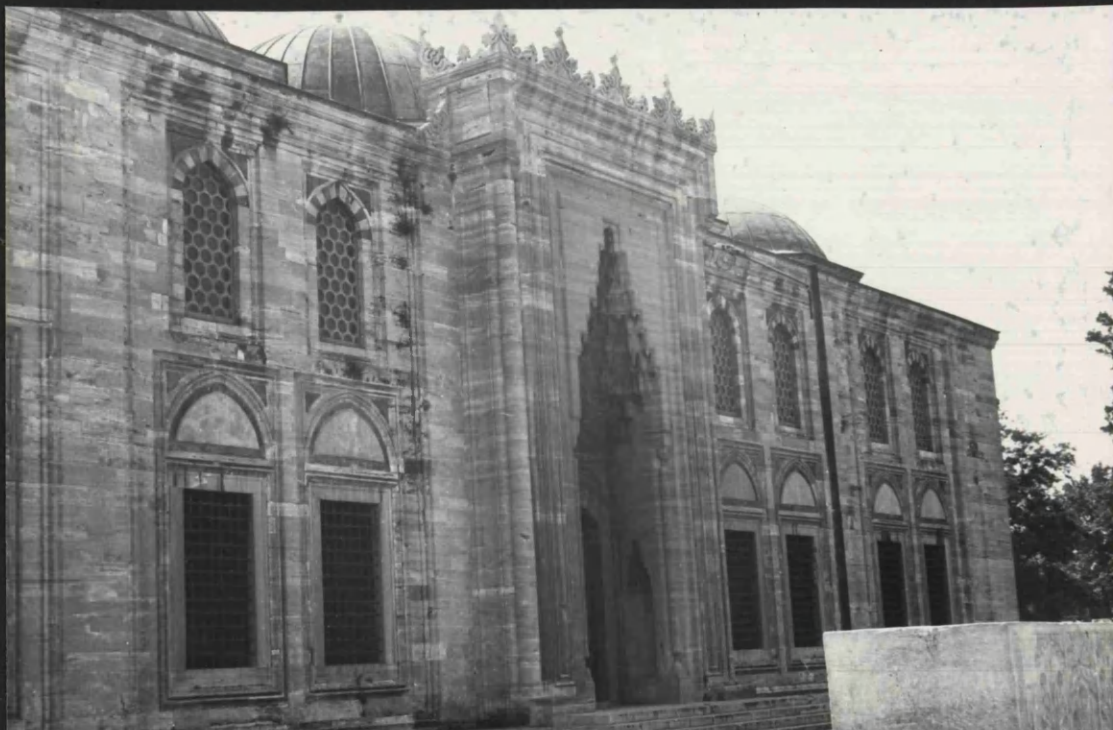
FIG. 23 THE NORTH WEST FACADE
