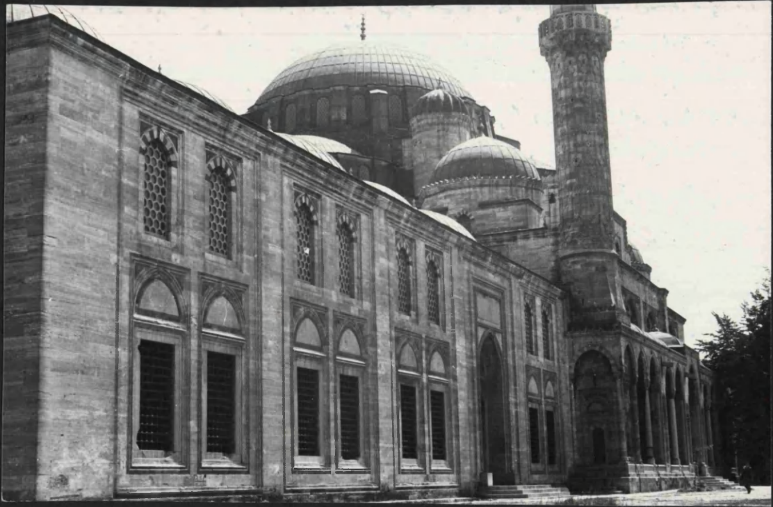
FIG. 18 THE SOUTH-WEST COURTYARD FAÇADE
