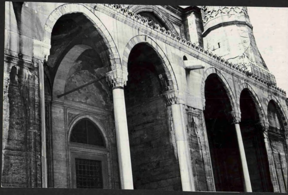
FIG. 28 THE PIERS AND COLUMNS OF NORTH-EAST LOGGIA
