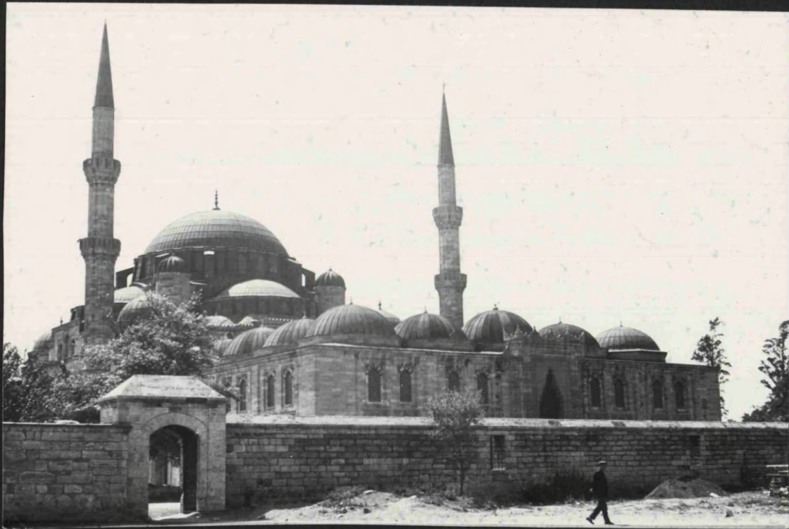
FIG. 22 THE NORTH WEST FACADE
