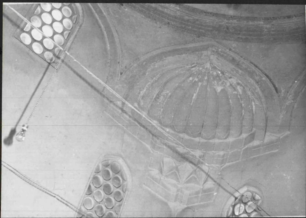
FIG. 112 THE SQUINCH OF THE READING ROOM
