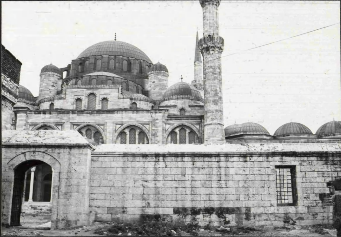
FIG. 63 THE NORTH-EAST FAÇADE OF THE CAMI
