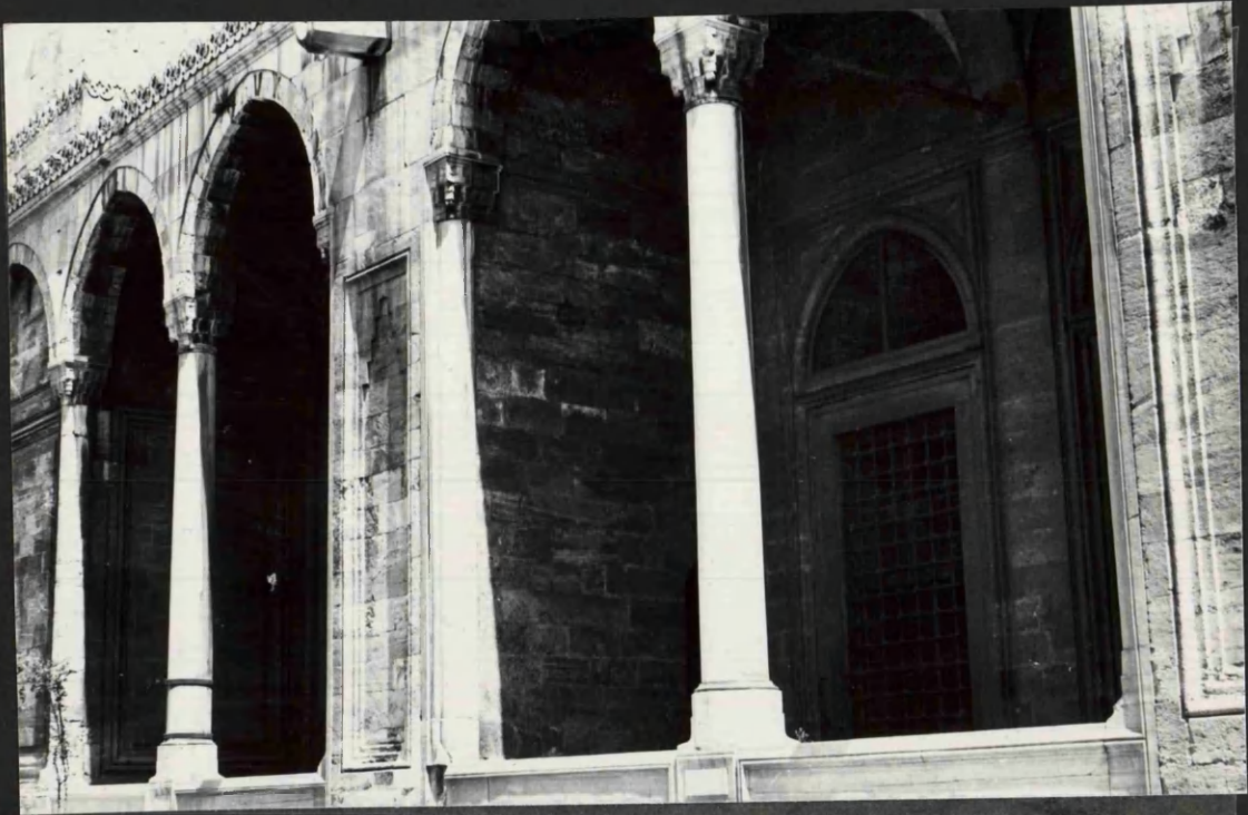
FIG. 7. THE SOUTH-WEST LOGGIA
