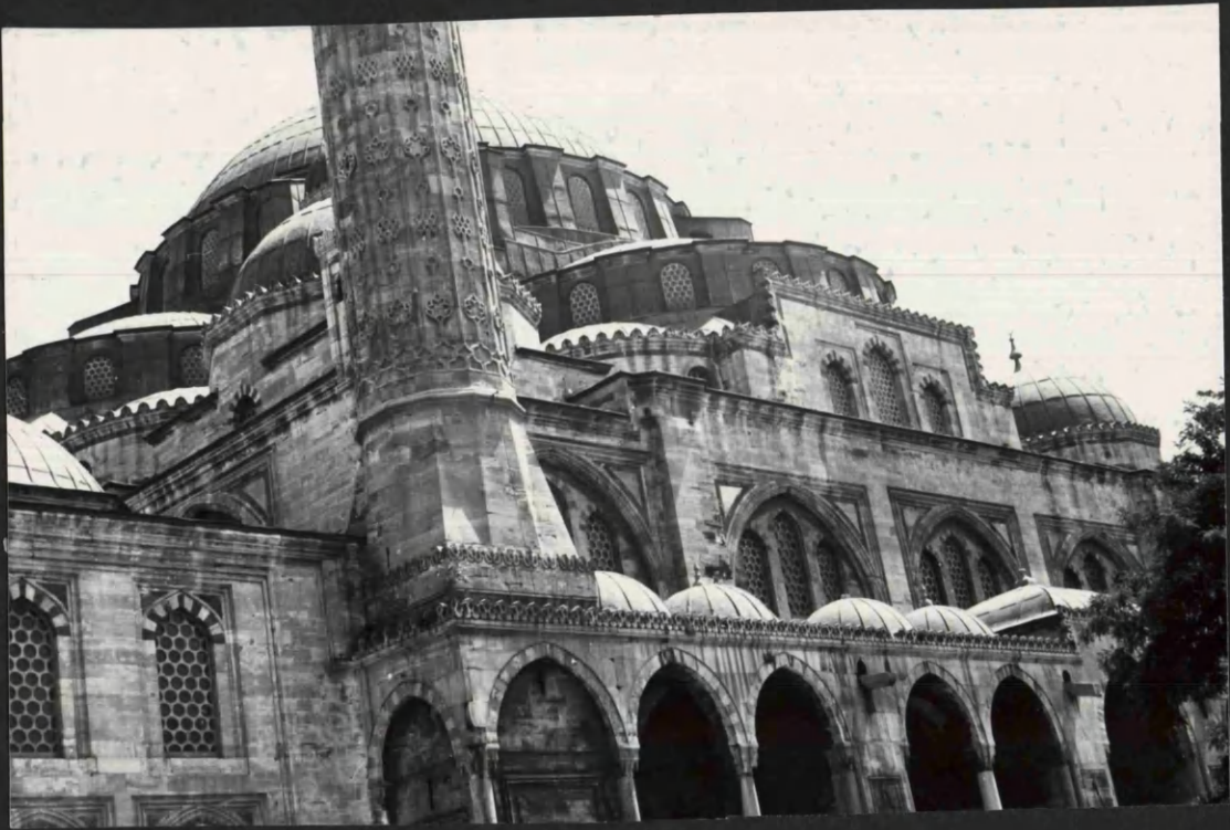
FIG. 10 THE SOUTH-WEST MINARET BASE
