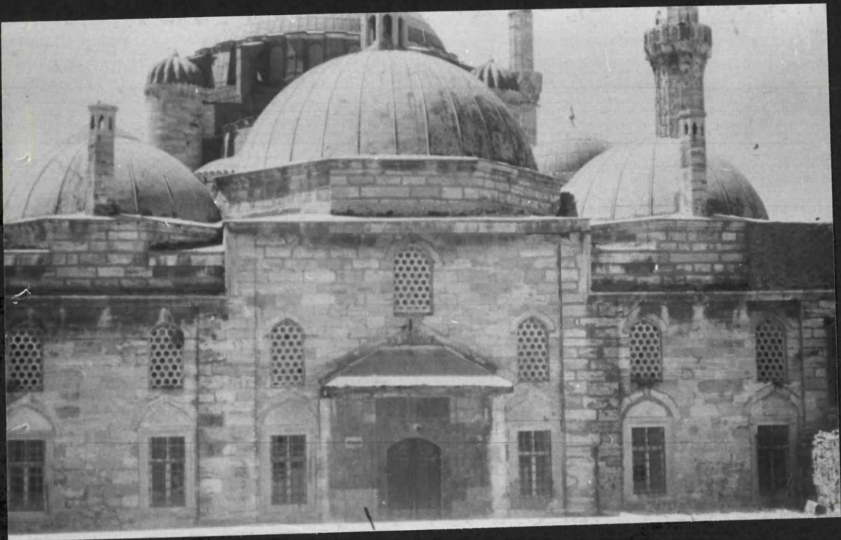
FIG. 114 THE FACADE OF THE TAPHANE
