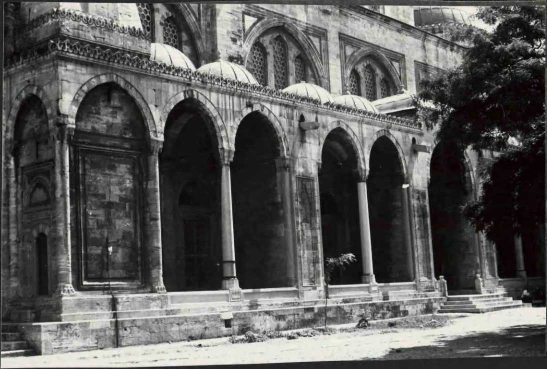
FIG. 6. THE SOUTH-WEST LOGGIA
