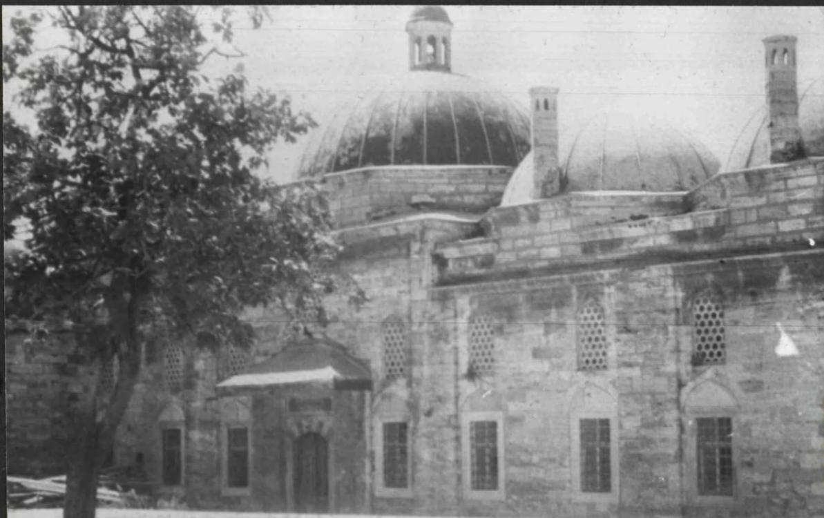
FIG. 115 THE FACADE OF THE TAPHANE
