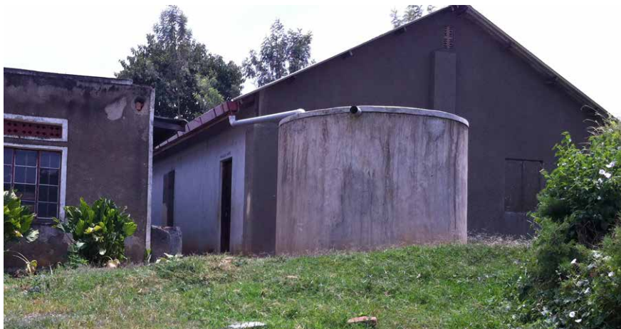
Rain water tank supplies water for 1,100 students
