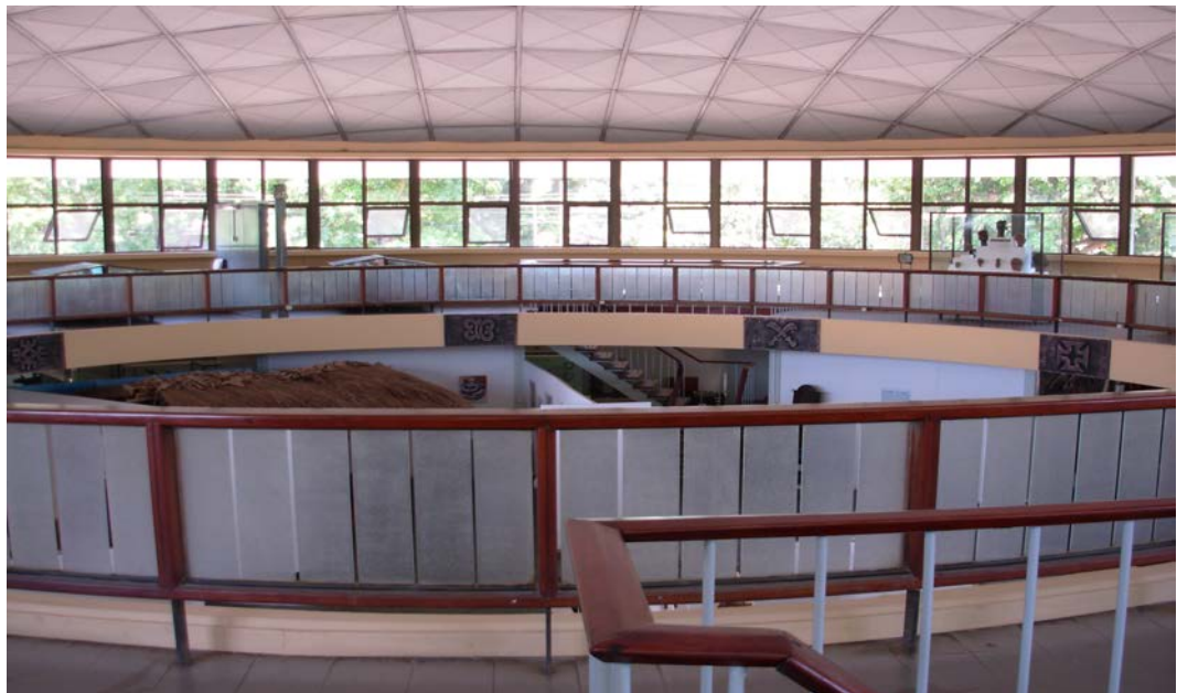
Figure 8: the circular galleries at the NMG (2007)
